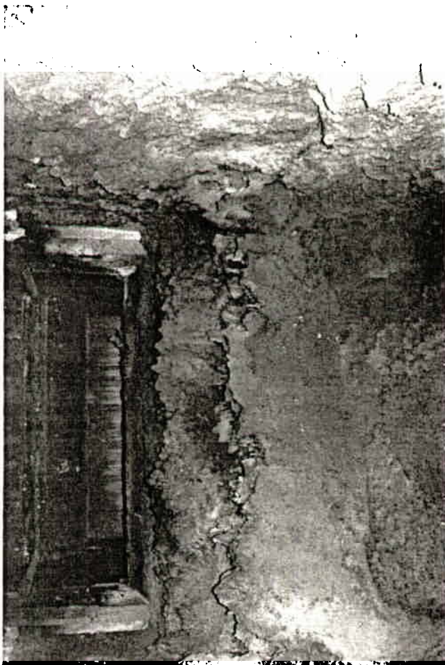
Figure. 4. Slag Build-up Over Secondary Air Nozzles.
